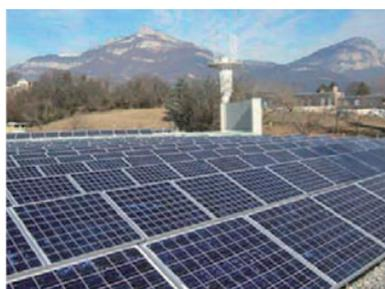
Fig. 9 - Installation mc-Si, 750kWc
